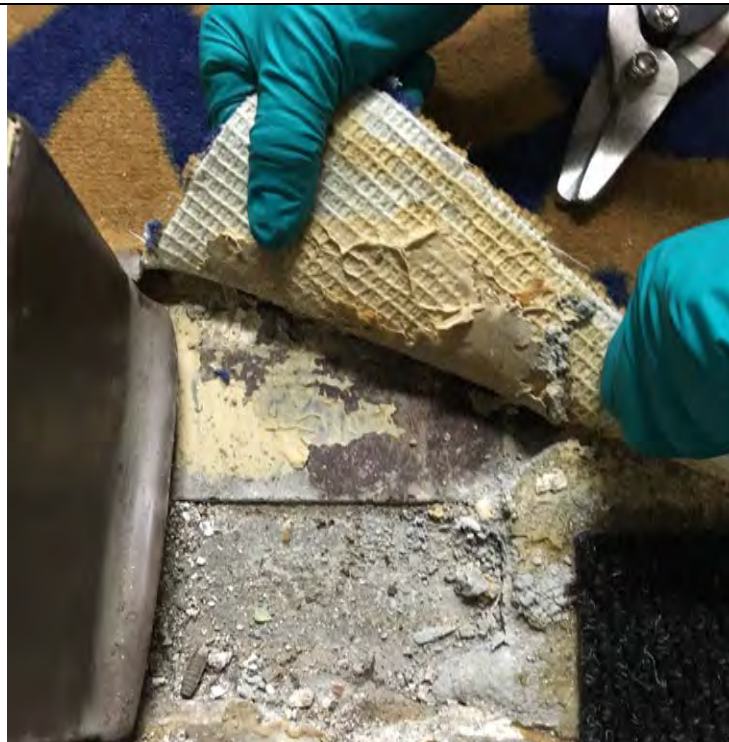
Photo #1 View of the asbestos containing red/brown vinyl floor tile (HA#12) and associated black mastic (HA#13) beneath the carpet in the reception area of the office building.
