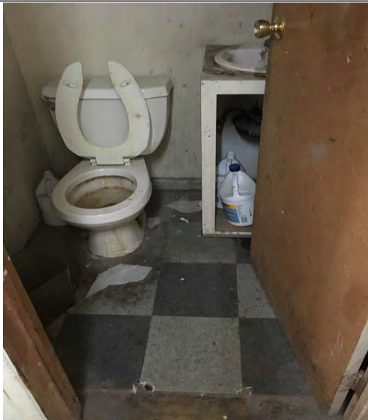
Photo #2 View of the asbestos containing black mastic beneath the vinyl floor tiles in the restroom of the storage building (HA#36).
