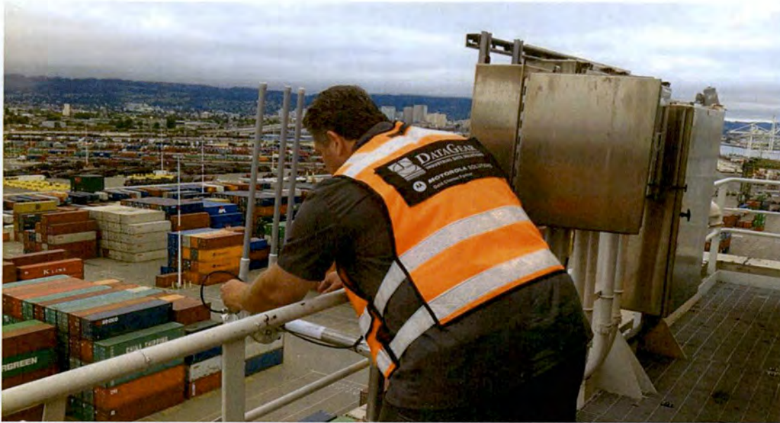
Motorola Wireless Link Installation Top of 300 foot Post Panamax Crane
