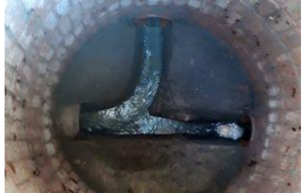
Manhole Before Install
