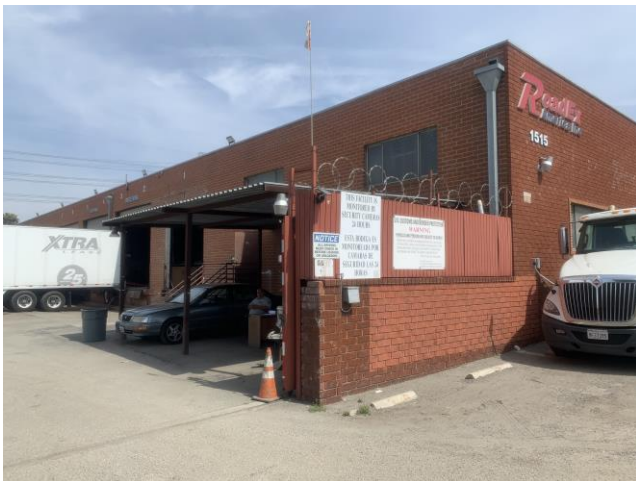
Photo 5: 1515 West 178 th East Elevation (NE)
