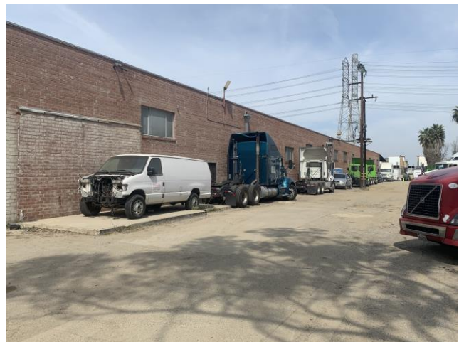
Photo 6: 1515 West 178 th East Elevation (NE)
