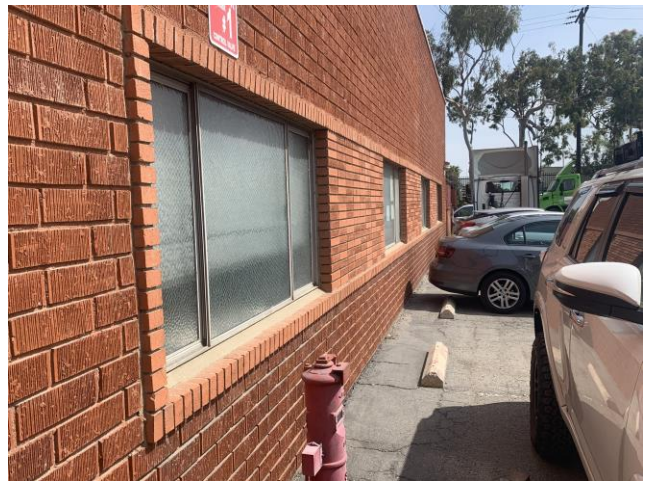
Photo 4: 1515 West 178 th West Elevation (NNW)
