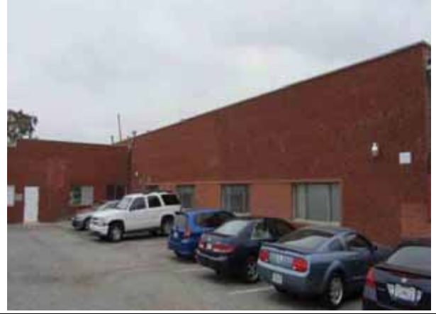
South side of building. View to the northwest.
