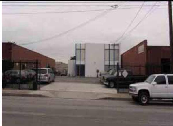
Southern adjacent property.
