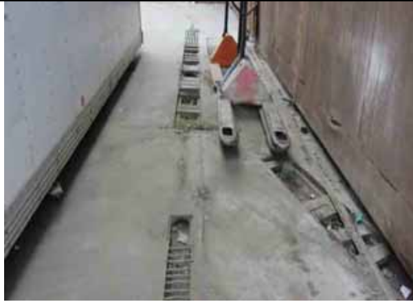
Trench drains on north side of building.
