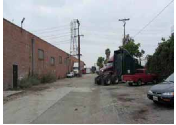
East side of building. View to the north.
