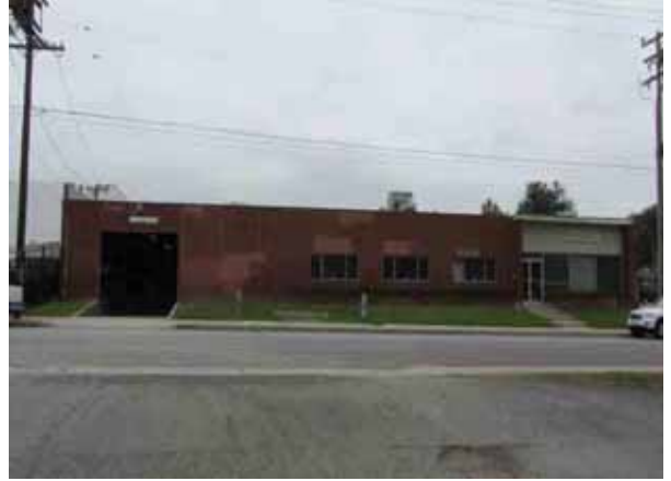
Southern adjacent property.
