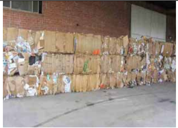
North side of building. View to the southwest.
