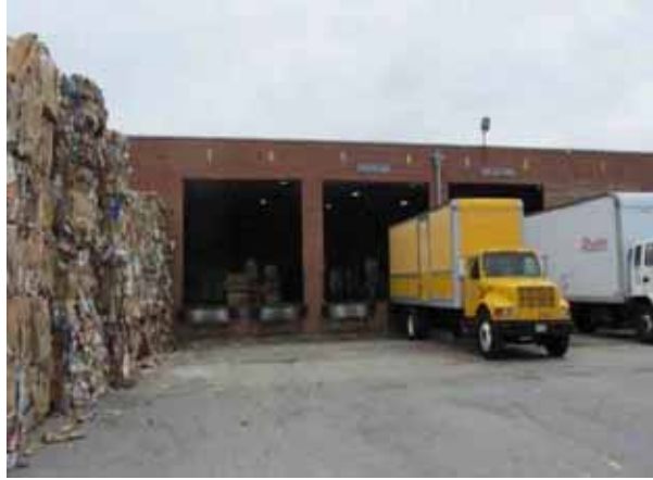
West side of building. View to the east.
