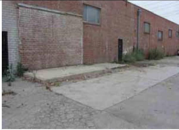
East side of building. View to the northwest.
