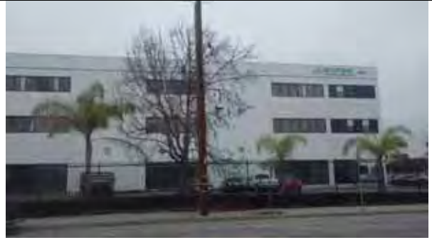
View of east adjacent property from south facing north
