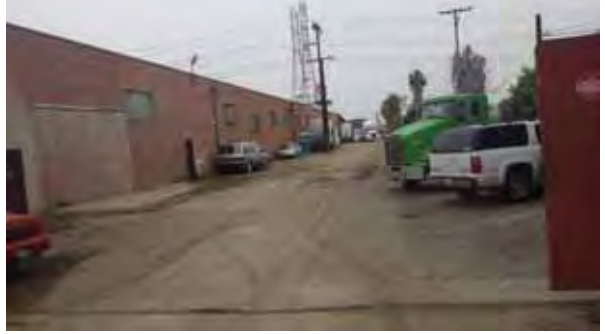
View of parking area west side of building
