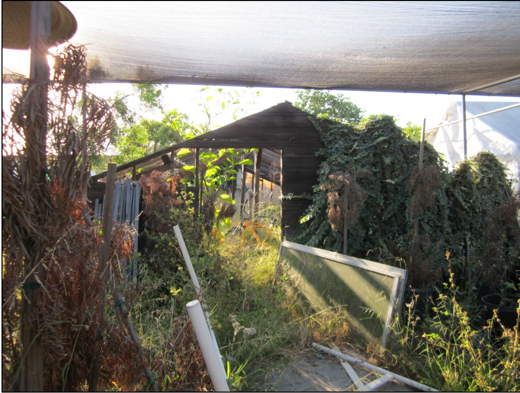
Figure 14. Shed/Greenhouse (APN: 6115-013-011), west façade
