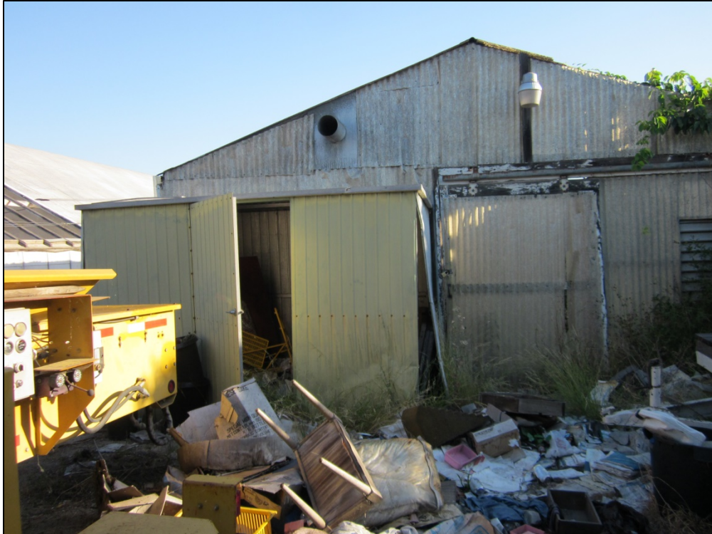
Figure 17. Large Shed (1343 W. 141 st Street), south elevation
