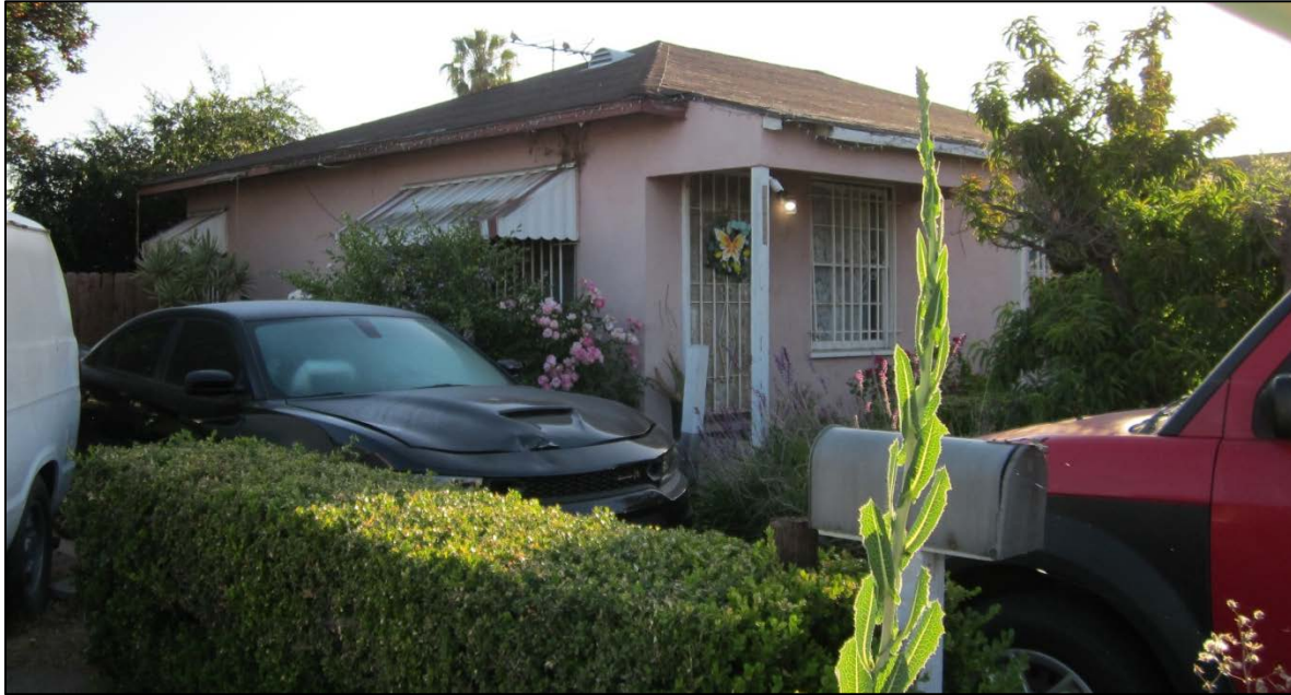
Figure 8. Single family residence (1335 W. 141 st Street), west elevation (left) south façade (right)
