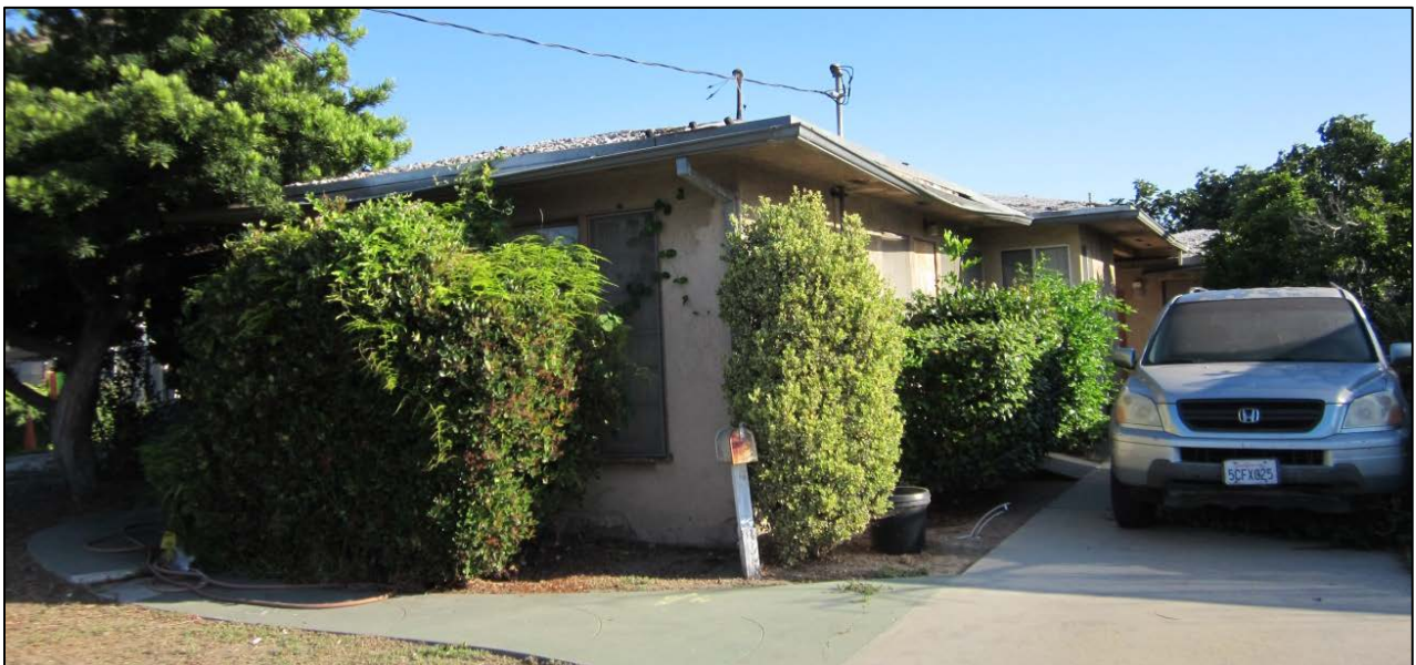
Figure 11. 1341 W. 141 st Street, South elevation (left) and east elevation (right)
