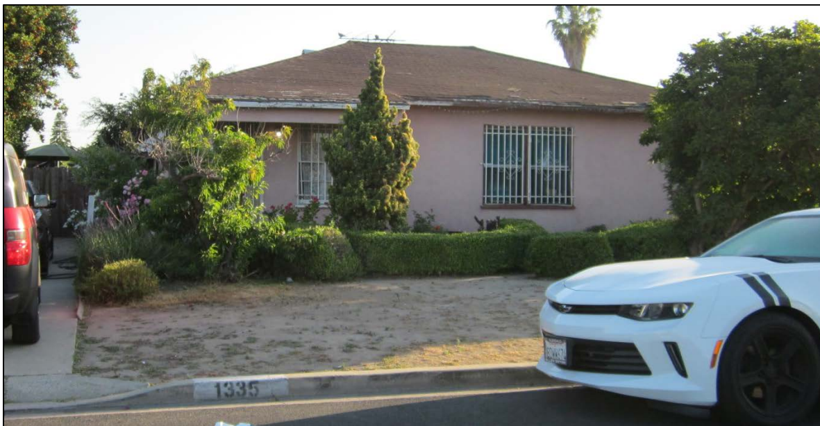
Figure 9. Single family residence (1335 W. 141 st Street) south façade
