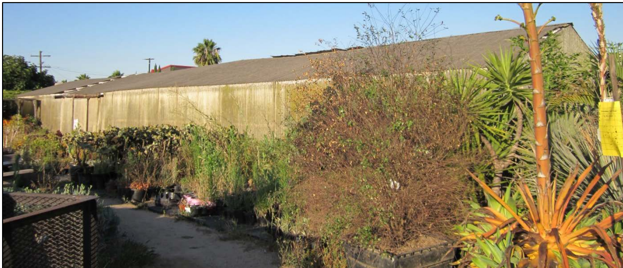
Figure 16. Large Shed (1343 W. 141 st Street), east elevation
