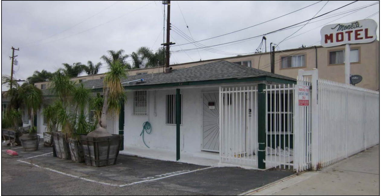
Figure 5. Moneta Motel, south elevation
