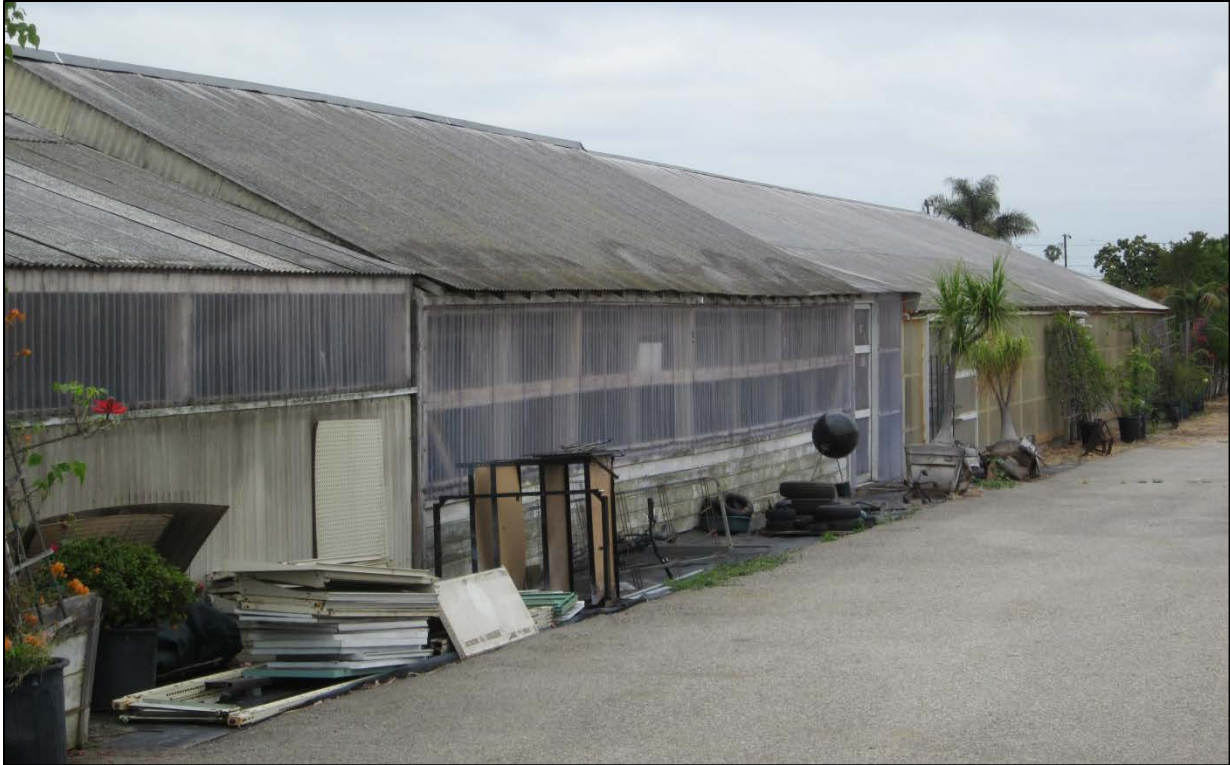
Figure 13. Green houses, north elevation
