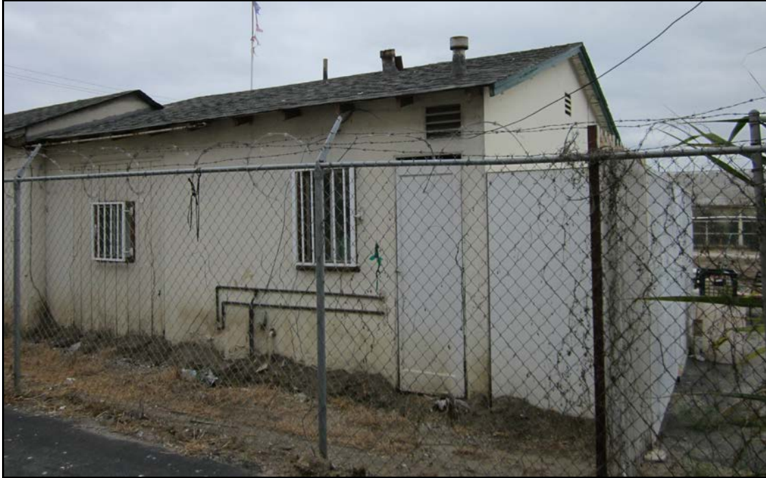
North elevation (rear of building) of honeymoon suite
