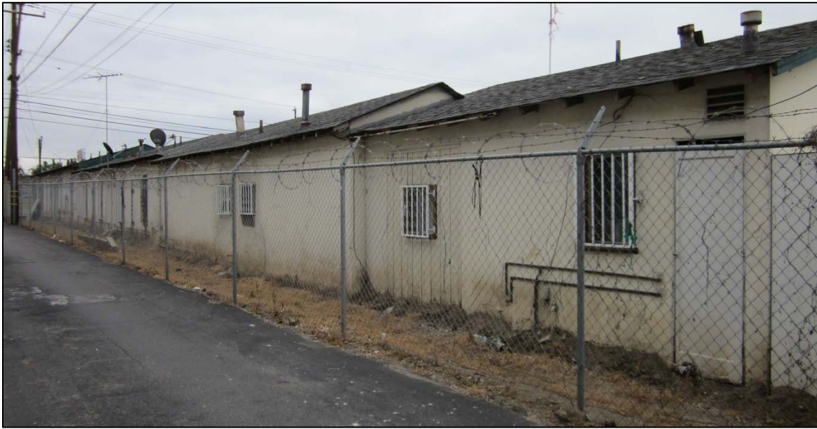
Figure 8. North elevation, looking southeast
