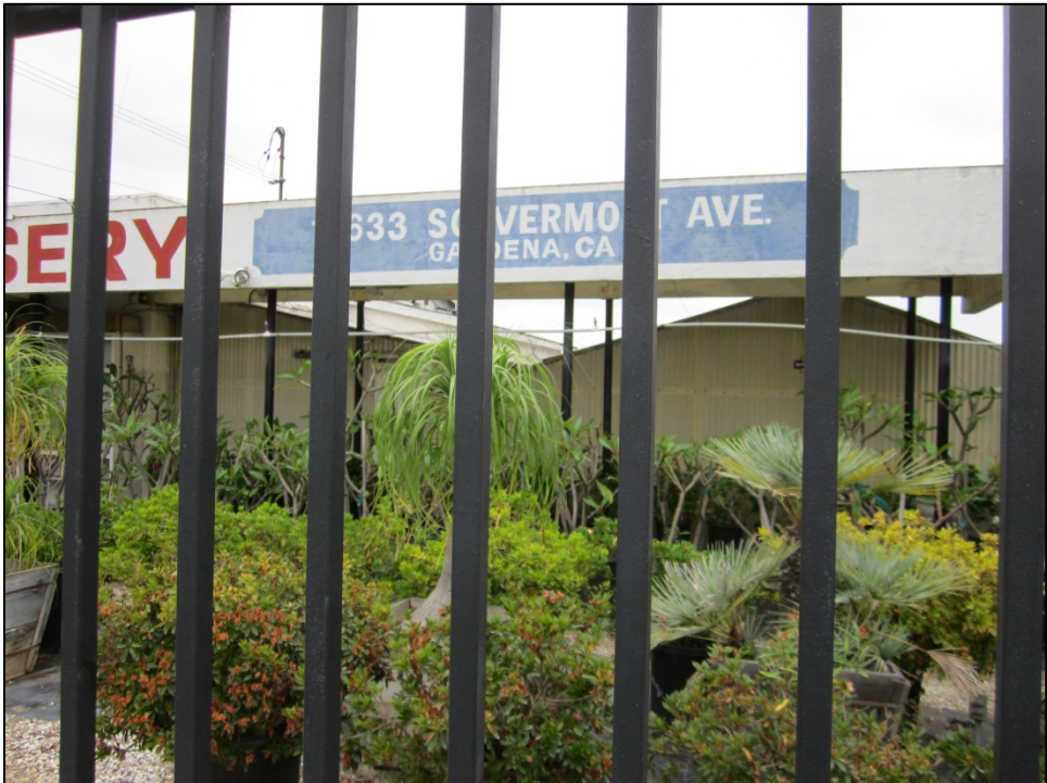
Figure 12. East elevation, twin gabled sheds/ greenhouses, facing west
