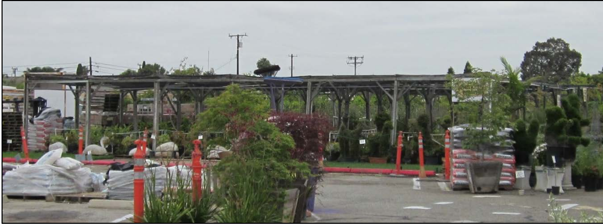
Figure 15. Wood framed shelter, located directly south of the main building
