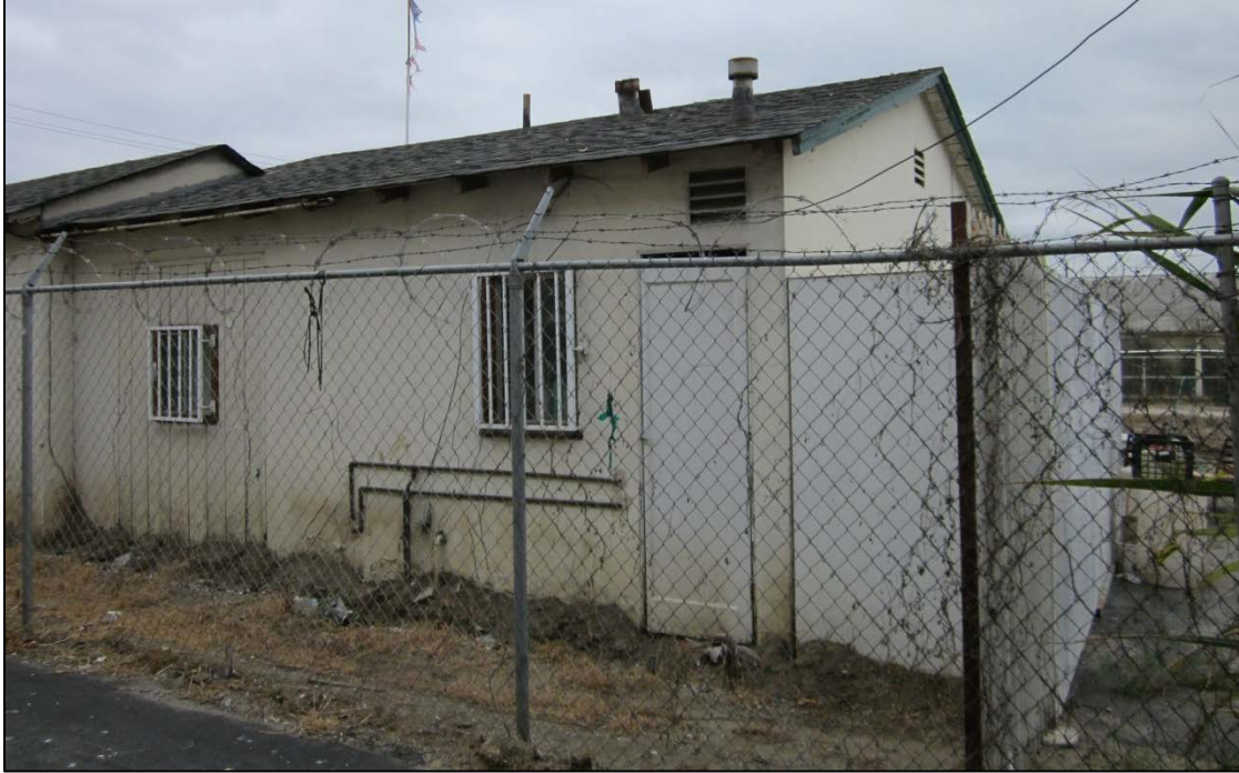
Figure 9. North elevation (rear of building) of honeymoon suite
