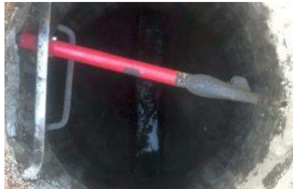
Manhole Before Install
