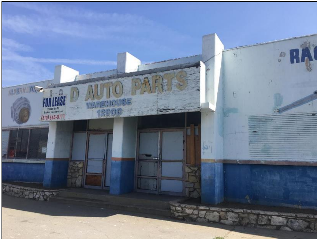
Figure 5. Detail of primary entrance, view northeast (SWCA, 2020).
