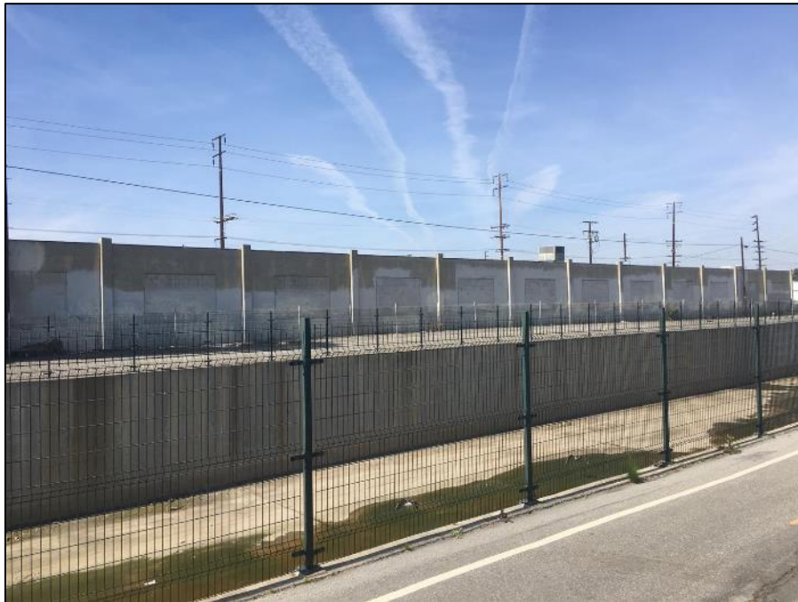
Figure 10. Overview of east (rear) façade, view northwest (SWCA, 2020).
