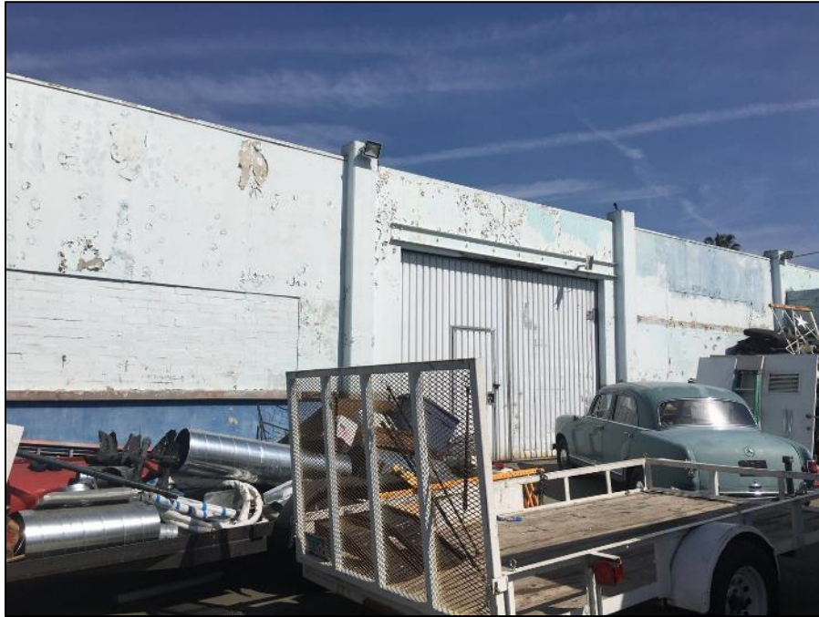
Figure 8. West end of south façade, view northeast (SWCA, 2020).
