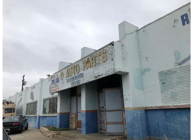
View of the Property, facing northeast
