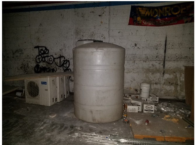
View of an empty 1,000-gallon AST
