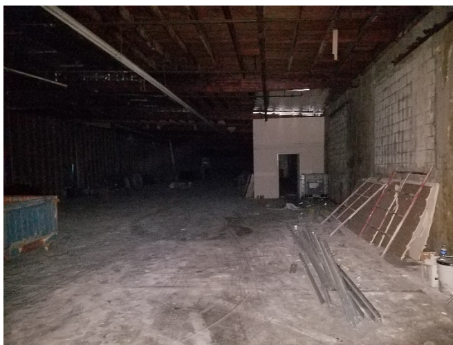
View of the interior east side of the building, facing north
