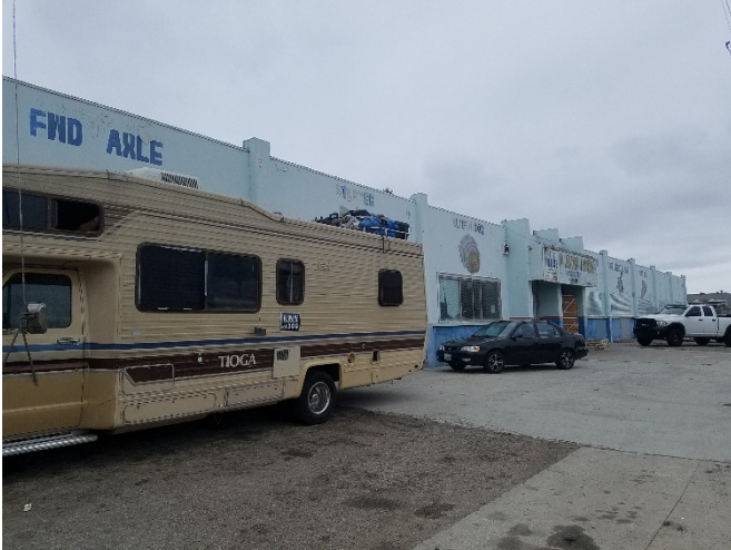
View of the Property, facing southeast
