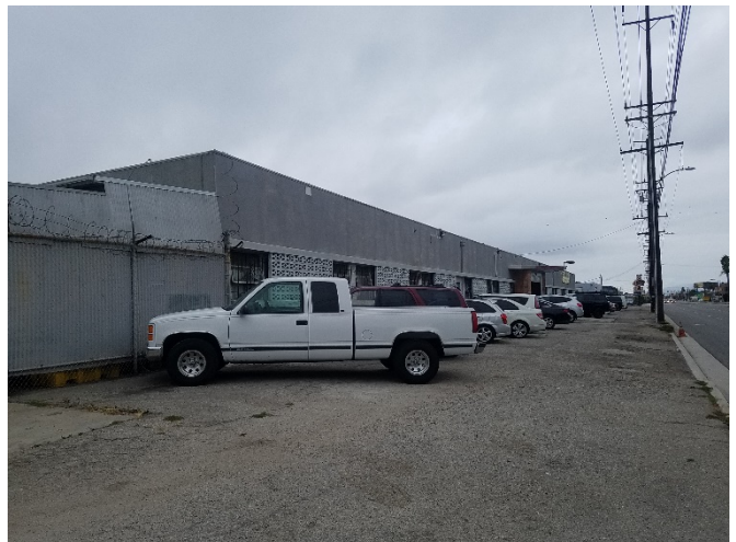
View of the south adjoining site
