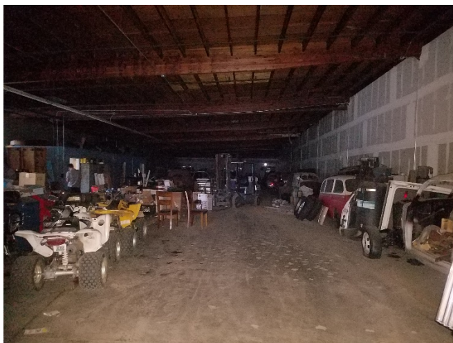
View of the interior west side of the building, facing north
