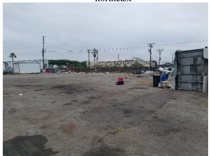
View of de minimis staining on the northern parking lot
