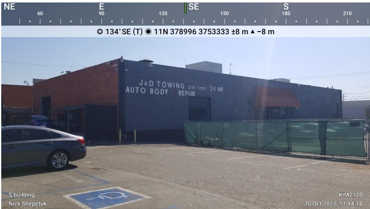
Photo 2: Industrial Building at 13130 Western Avenue
