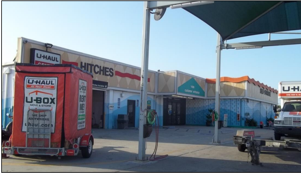
Figure 6. Main Storage, northern half of west façade
