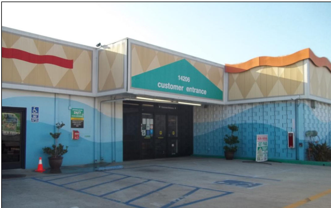
2. Portion of west façade of 14206 Van Ness Avenue
