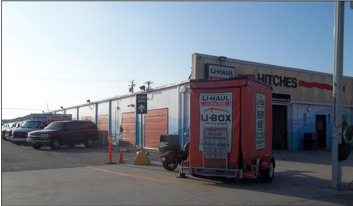
1. North elevation (left) and west façade (right); 14206 Van Ness Avenue
