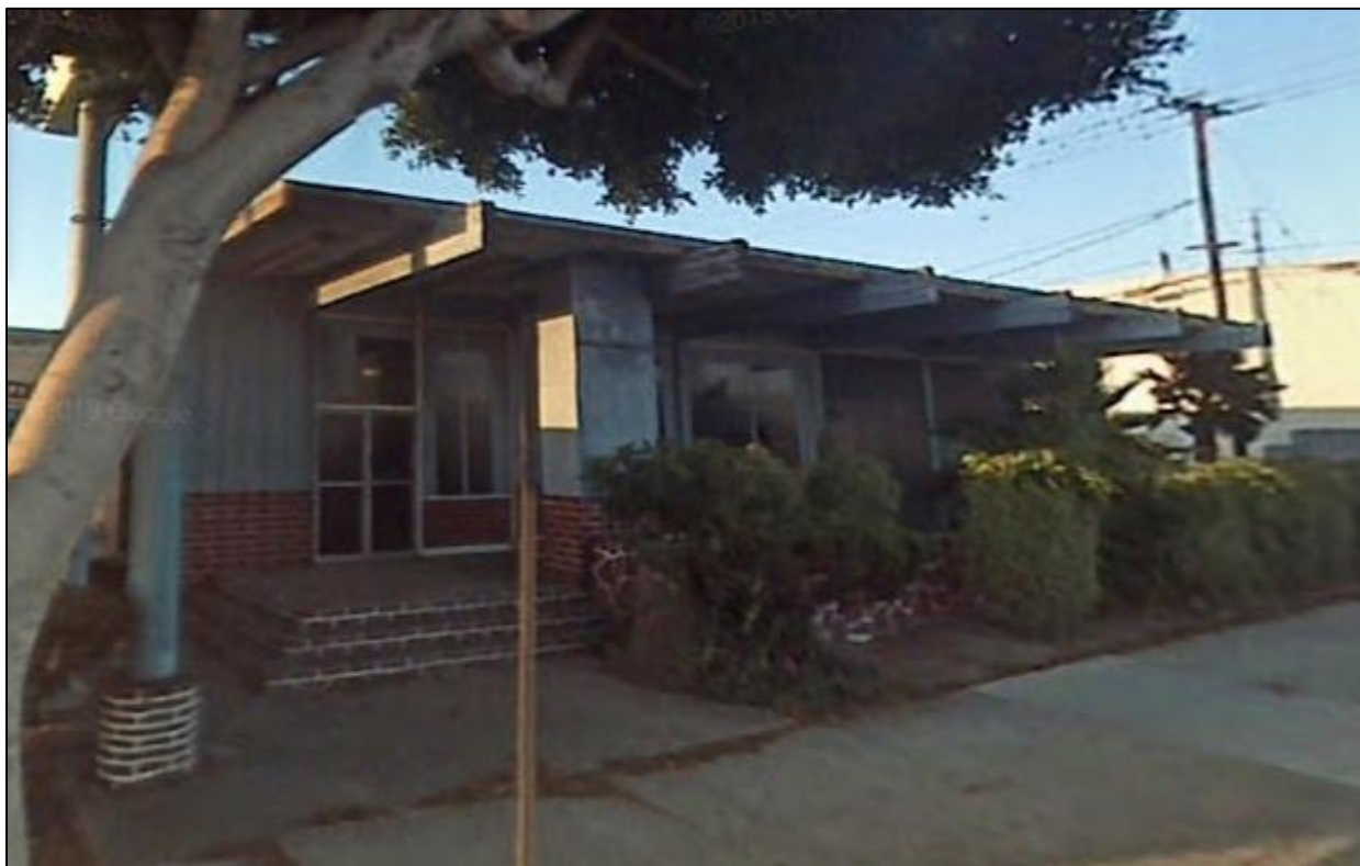
2145 Rosecrans Avenue, south façade, facing northeast (Google Street View 2007)
