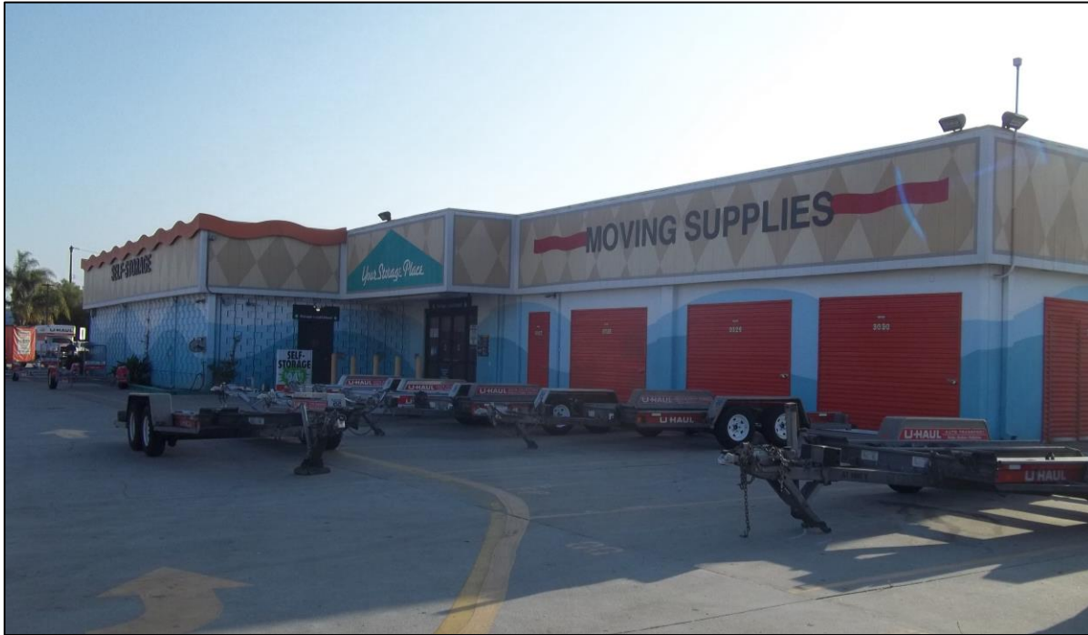
3. Portion of west façade (left) and portion of south elevation (right) of 14206 Van Ness Avenue
