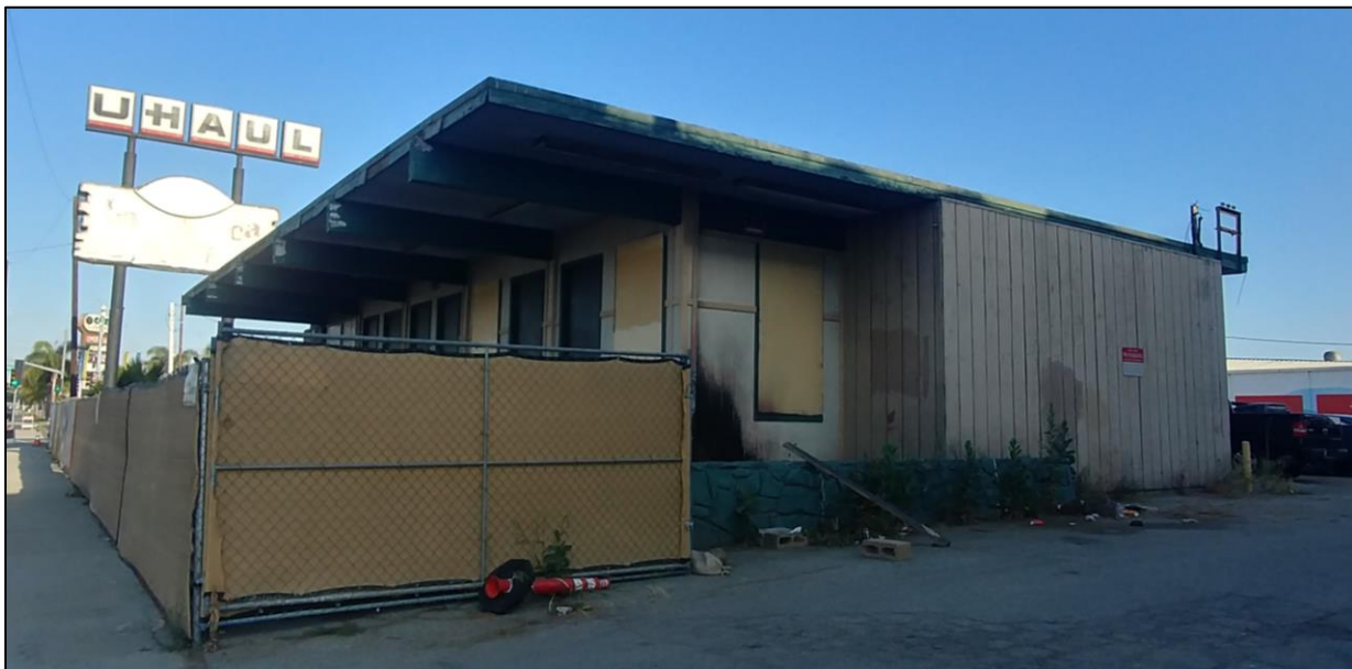
South façade (left) and east elevation (right); taken June 2021
