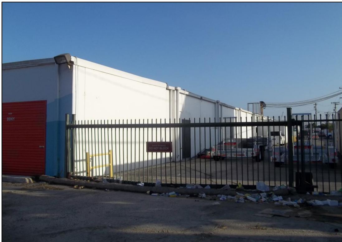
5. Portion of south elevation (left) and east elevation (right) of 14206 Van Ness Avenue
