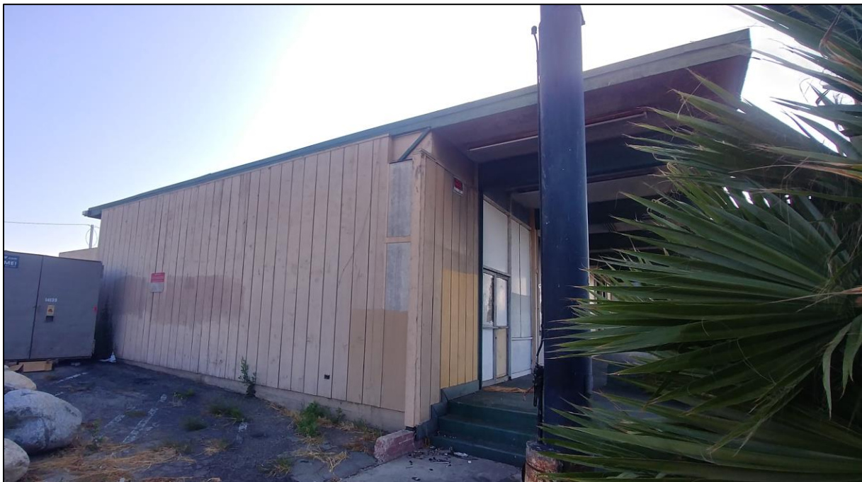
West elevation (left) and south façade (right); taken June 2021
