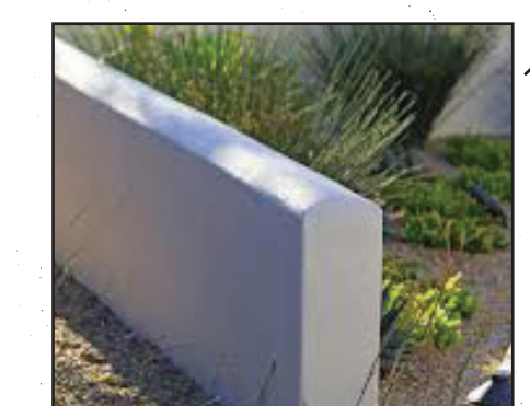
Stucco pony wall
