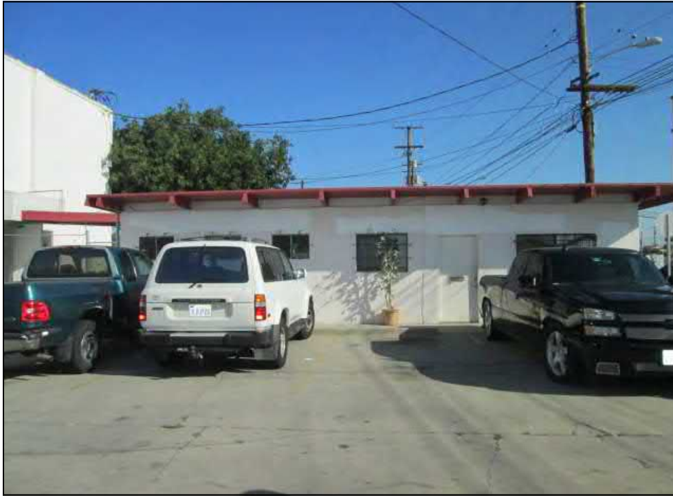
Photo 1: View of the office structure at the subject property (16829 South Normandie Avenue).
