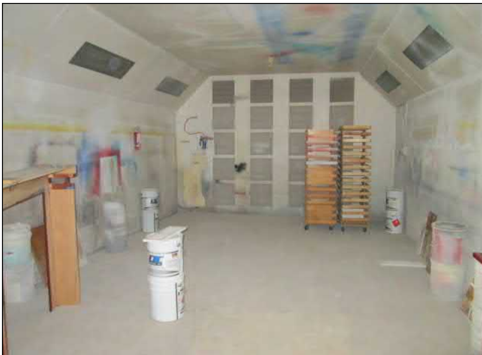
Photo 20: Interior view of the spray booth.
