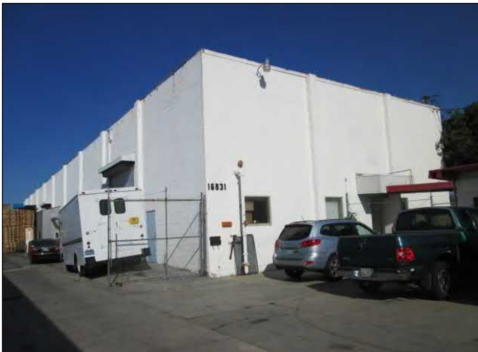
Photo 2: View of the industrial structure at the subject property (16831 South Normandie Avenue).
