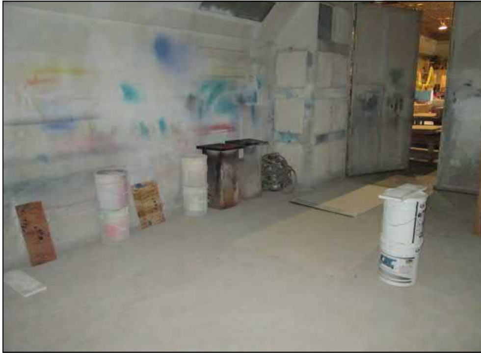
Photo 21: Additional view of the spray booth.
