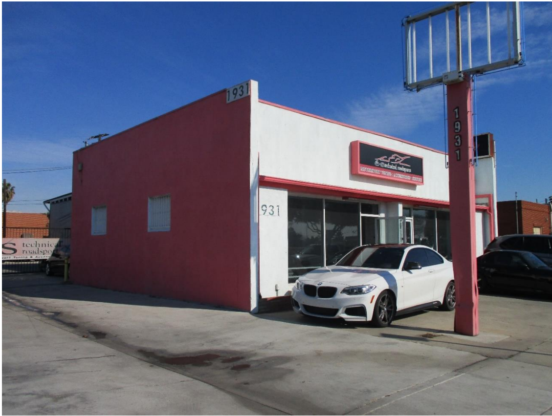
Figure 11. Overview of 1931 West Artesia Boulevard Looking Northeast (1/8/2019, IMG_1733)
