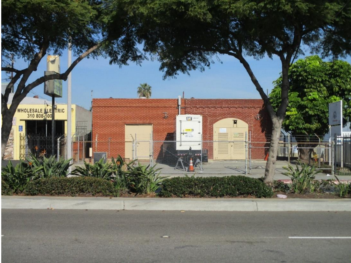
Figure 9. Overview of Main (South) Elevation, with 1928 Original Pumping Plant on right, and 1960 Addition on Left (1/8/2019, IMG_01744)
