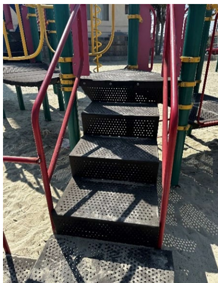
Play Structure Stairway
