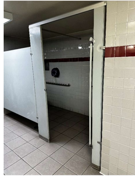
First Floor Women's Restroom Toilet
