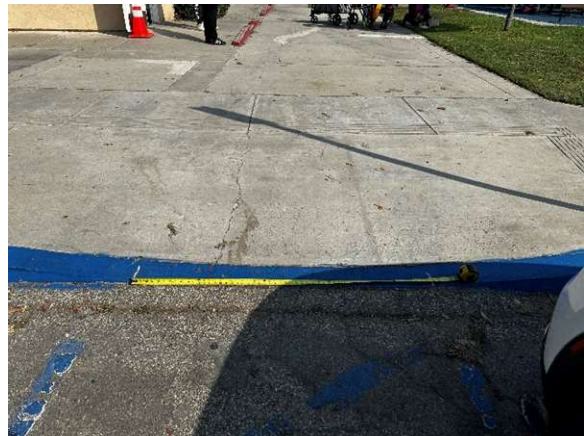
Curb Ramp at Parking Spaces 4 & 5
