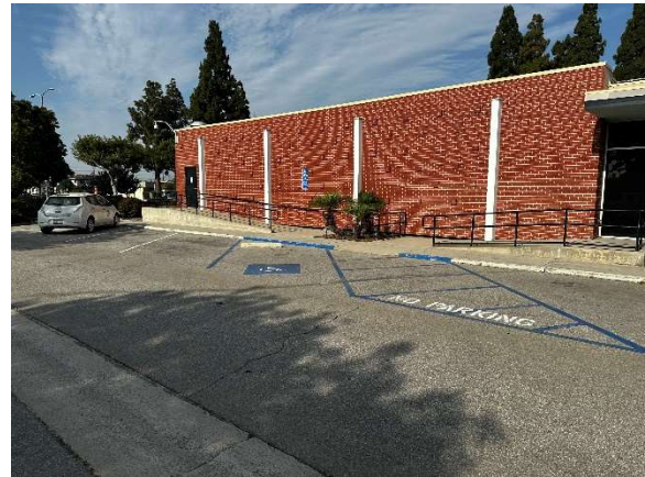
Parking Space 5 and Access Aisle 5
