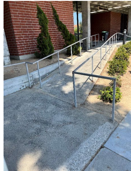
Office Entry Ramp
