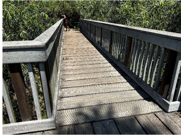
Bridge to Overlook
