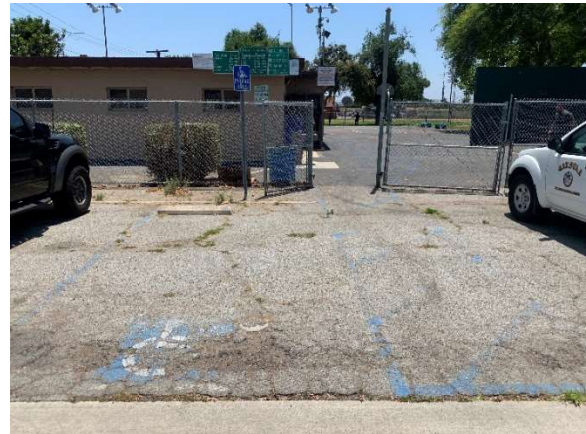
Existing Accessible Parking Space
