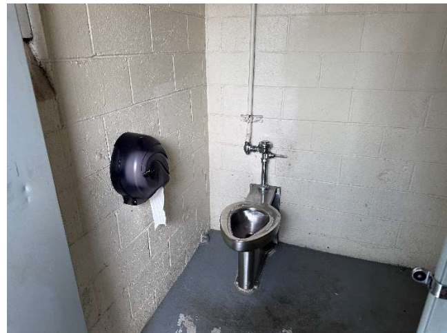
Women's Accessible Toilet Stall
