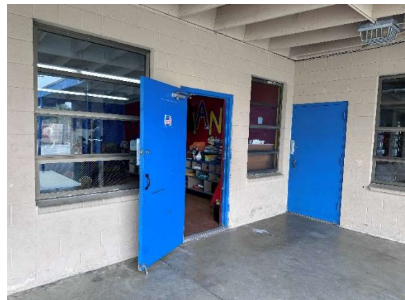
Classrooms 1 & 2 Entry Doors
