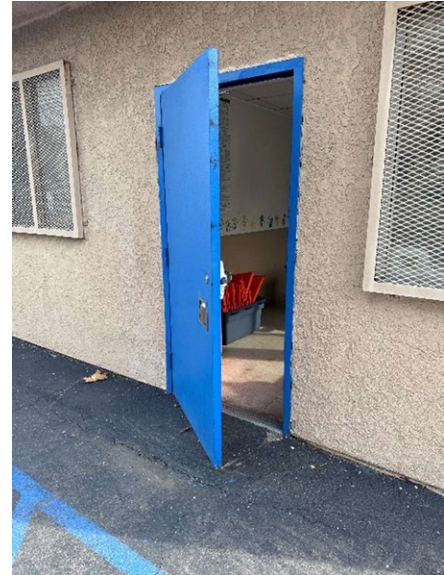
Door 1: Office Entry Door
