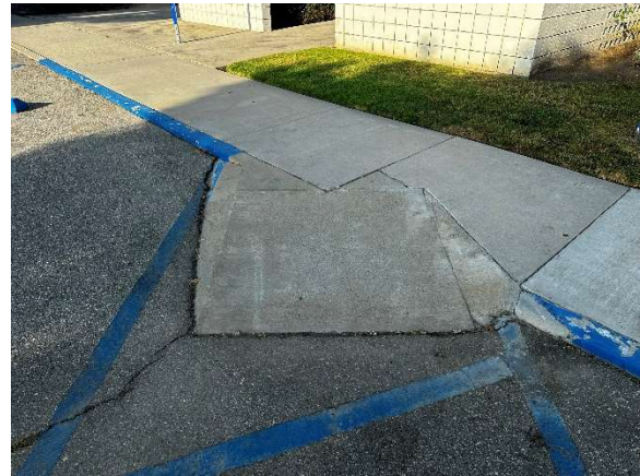
Built-up ramp in Access Aisle 1-2
