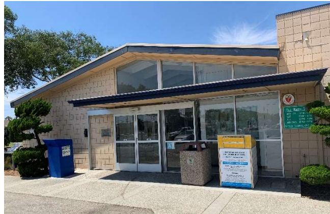
Recreation Building Main Entrance
