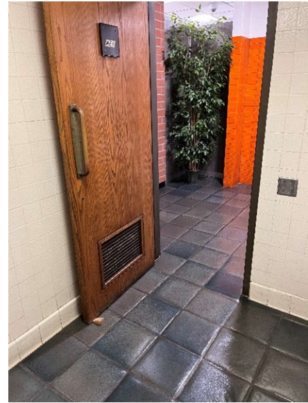
Men's Restroom Entry
