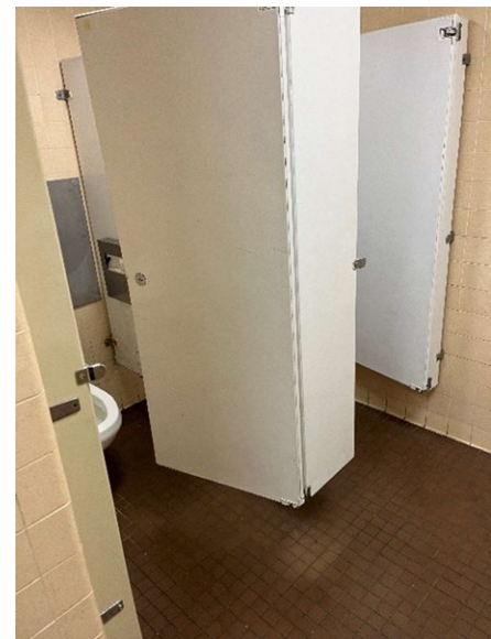
Men's Toilet Compartments
