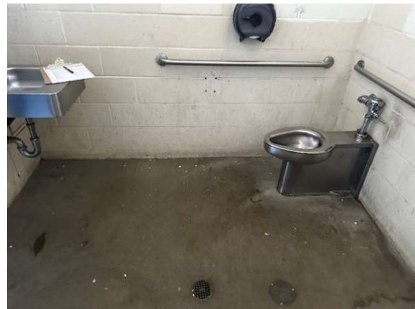
Restroom Building Interior
