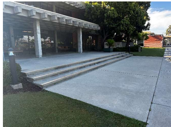
Main Entry Stairs
