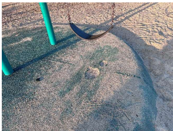
Worn Padded Surface at Belt Swings
