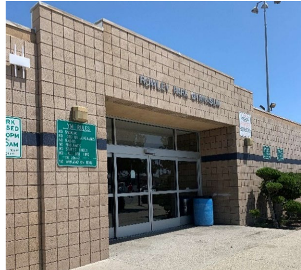
Rowley Gymnasium Entrance
