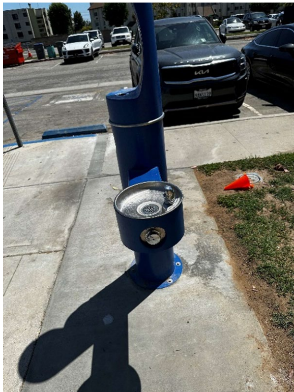
New Drinking Fountain and Water Bottle Filling Station
