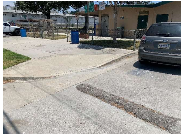
Halldale Avenue Pedestrian Entry
