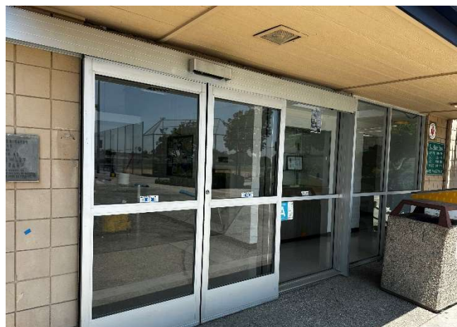
Recreation Building Entry Door
