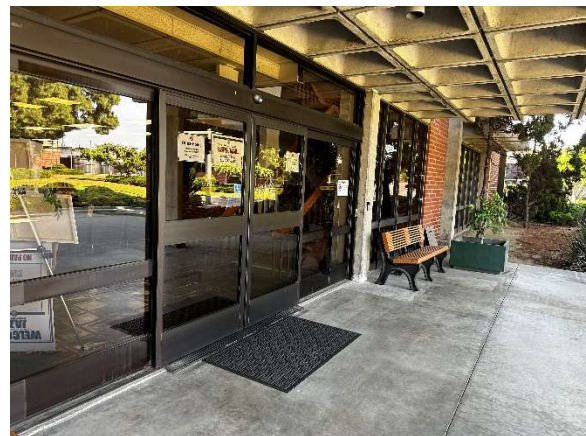
Main Entry Door
