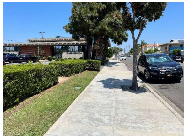
Public Sidewalk at W. 162 nd Street
