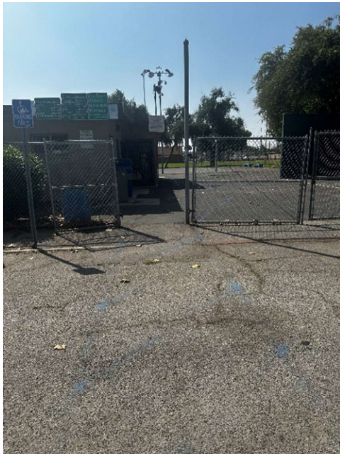
Main Entry Gate
