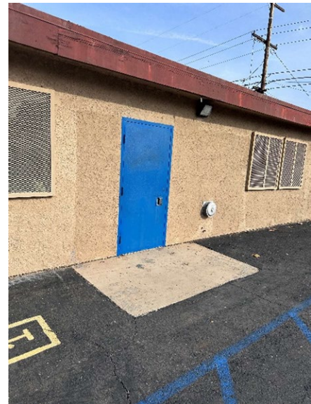
Door 2: Secondary Exit Door
