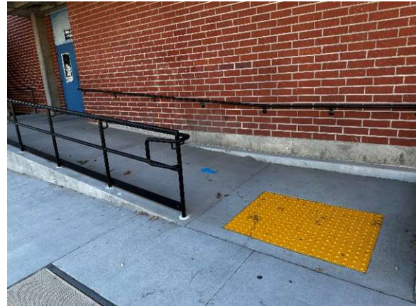
Gym Entry Ramp
