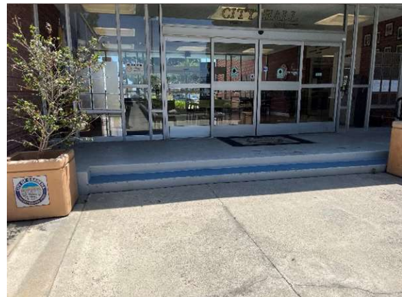
Stair2 and Door 2
