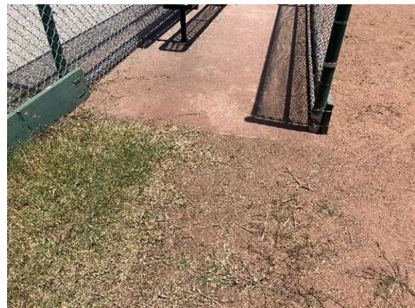
Dugout Surface Transition
