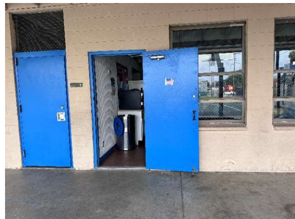
Classroom 1 Entry Door
