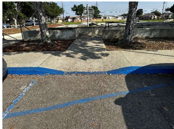
Curb Ramp at Parking Spaces 2 & 3
