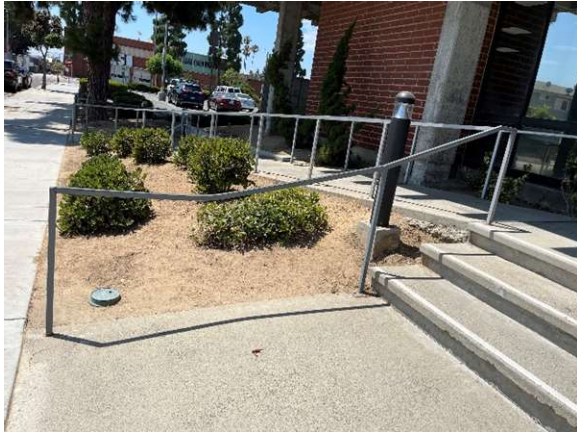
Office Entry Stairs
