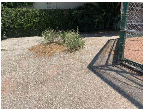
Paved Area behind Backstop
