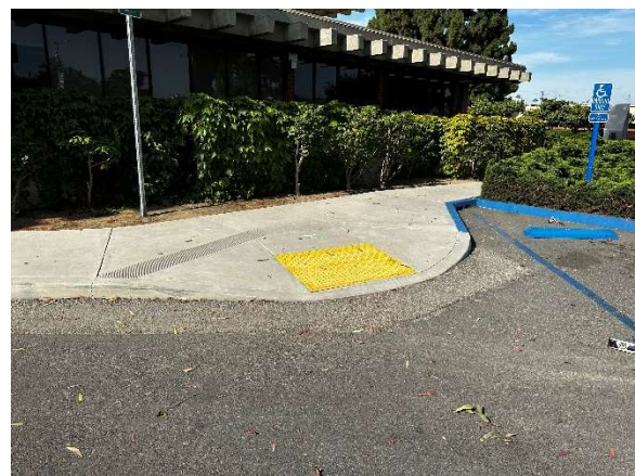
Curb Ramp at Accessible Parking
