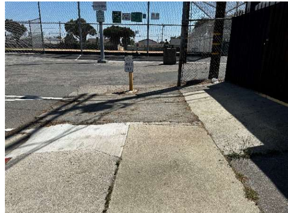
Sidewalk Entrance at 154th Place
