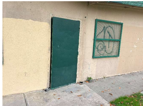
Rear Exit-Only Door
