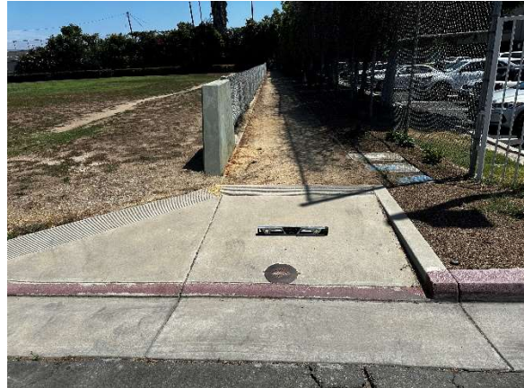
Curb Ramp Approach
