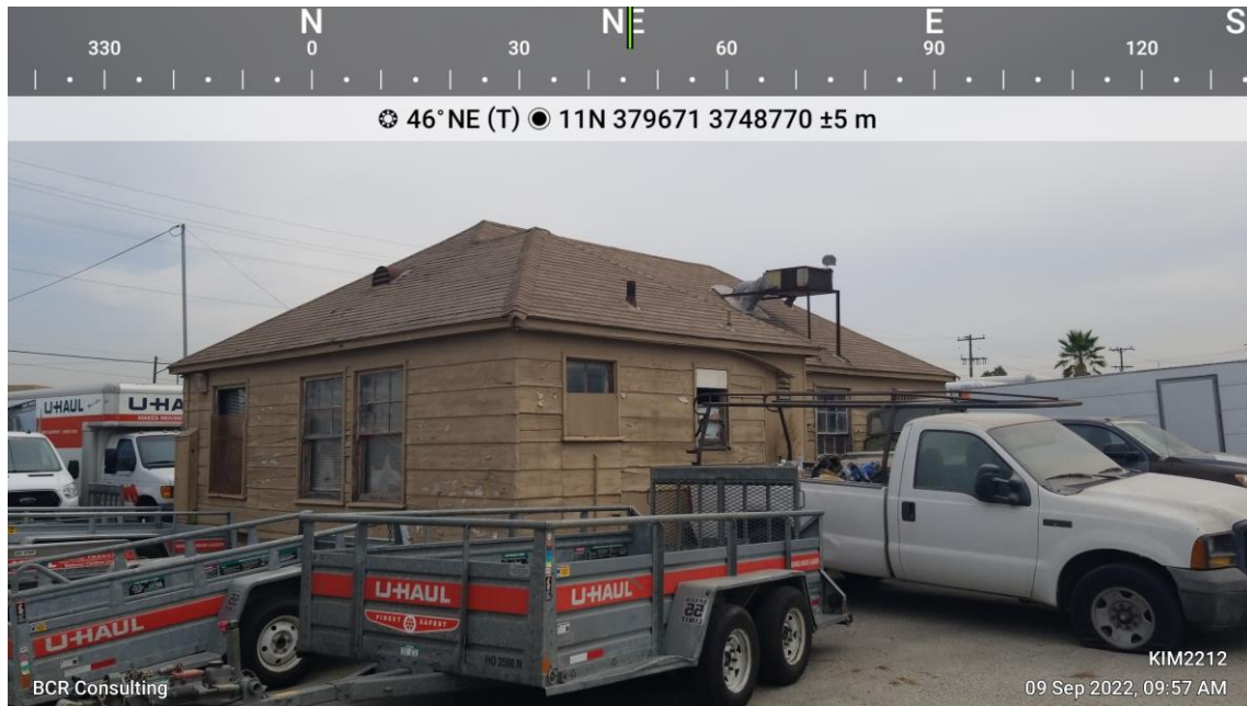
Photo 2: 1450 Artesia Blvd Building A, Southwest Corner (View Northeast)
