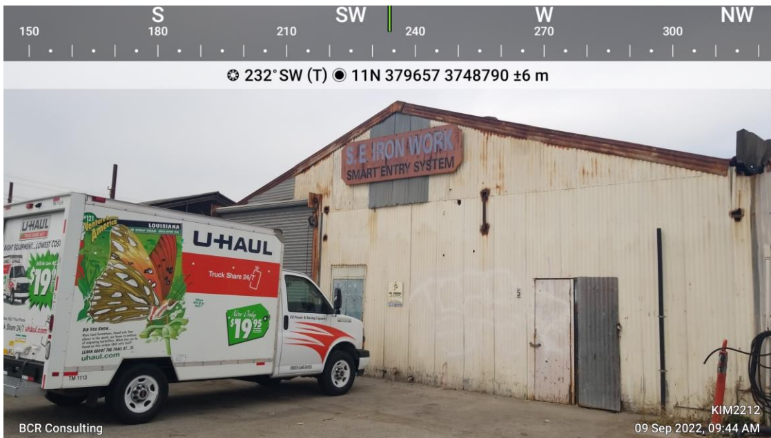
Photo 3: 1450 Artesia Blvd, Building B (View Southwest)
