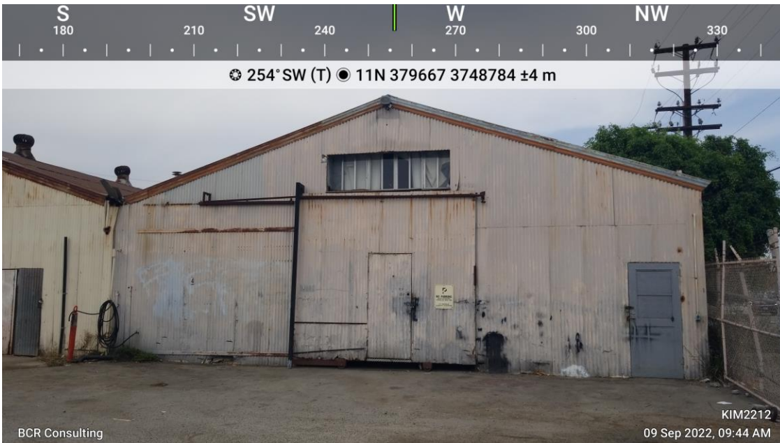
Photo 4: 1450 Artesia Blvd, Building B (View West)
