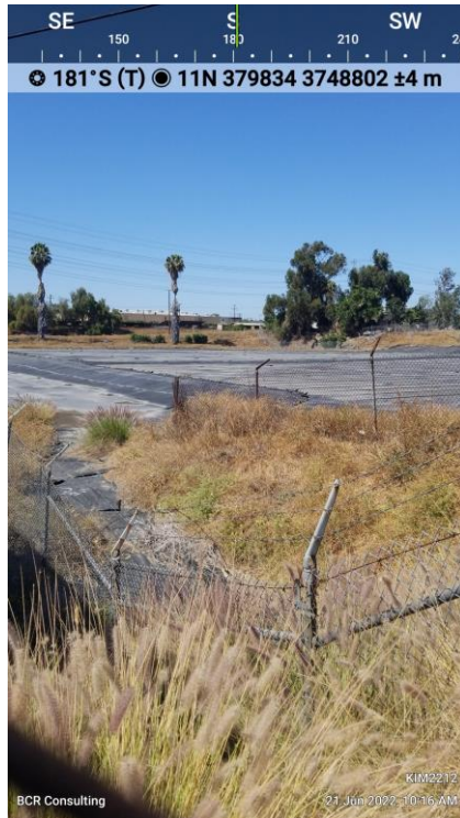
Photo 1: Petroleum Dump Site at 1450 Artesia Blvd (View S)
