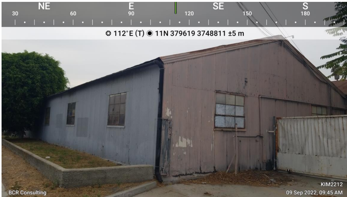
Photo 5: 1450 Artesia Blvd, Building B (View East)
