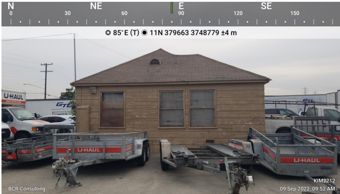
Photo 1: 1450 Artesia Blvd Building A, West Elevation (View East)
