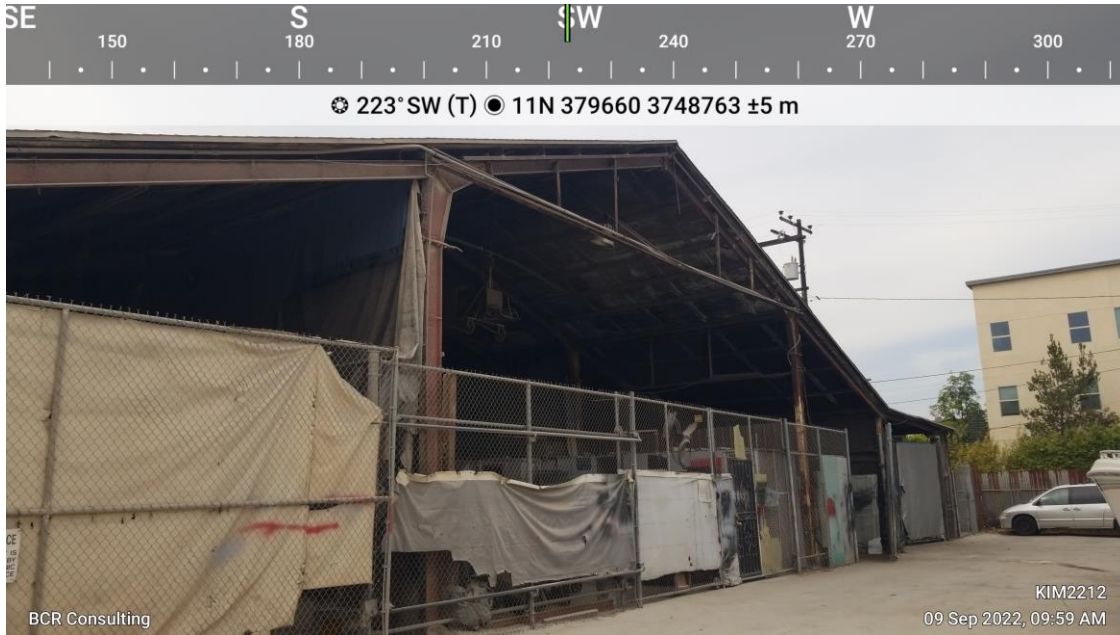
Photo 7: 1450 Artesia Blvd, Building C (View Southwest)
