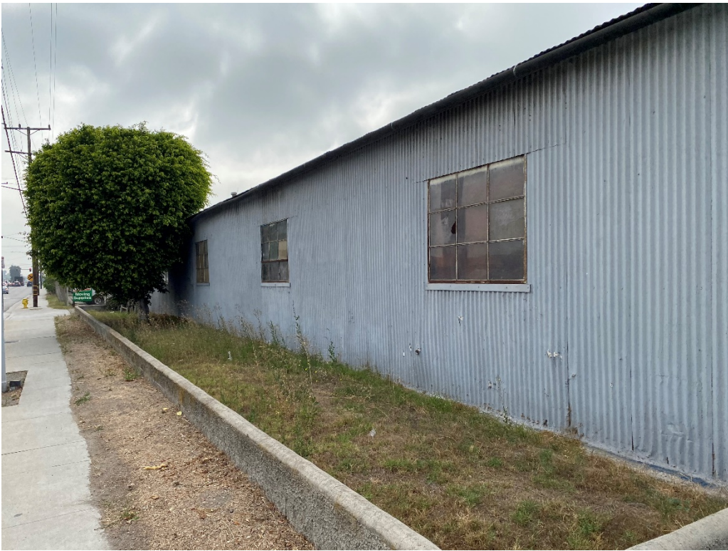
G-13. View from outside property facing side of metal building (9/3/2021).
