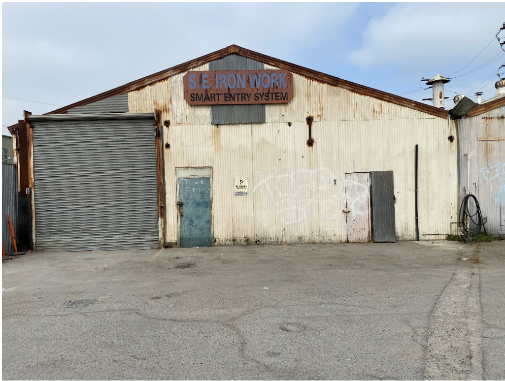
G-7. Directly in front of the SE iron work building (9/3/2021).
