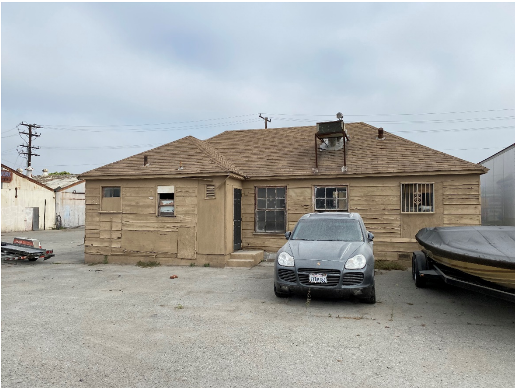
G-4. Back view of existing U-Haul office (9/3/2021).
