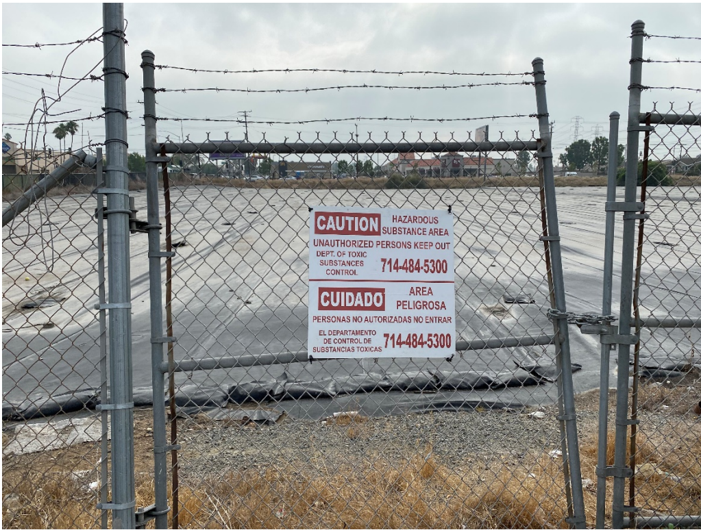
G-1. Entrance gate to hazardous waste area (9/3/2021).
