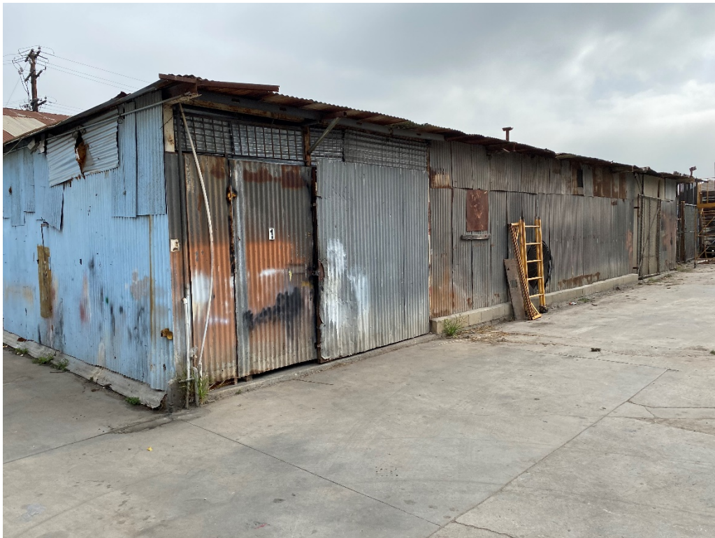
G-6. View from the back of the SE iron work building (9/3/2021).
