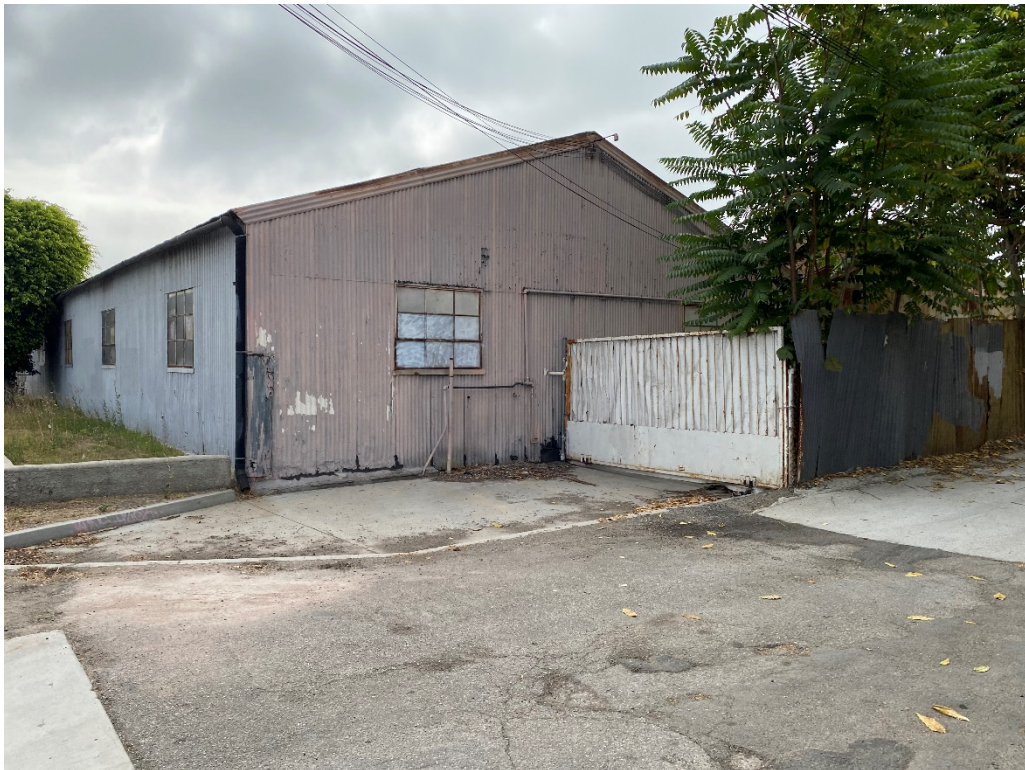
G-12. Back view of buildings and entrance gate (6/11/2021).
