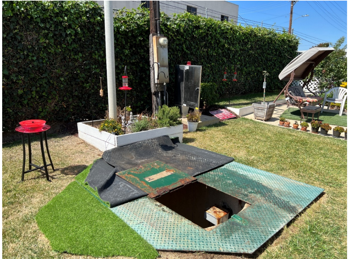
Figure 1.3 Lift Station Location
