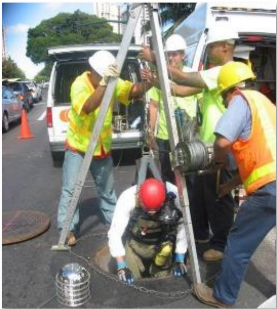
Photo 2-1. Confined Space Entry
