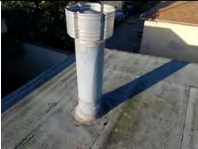
Photo 1: pump house roof and penetration mastic
