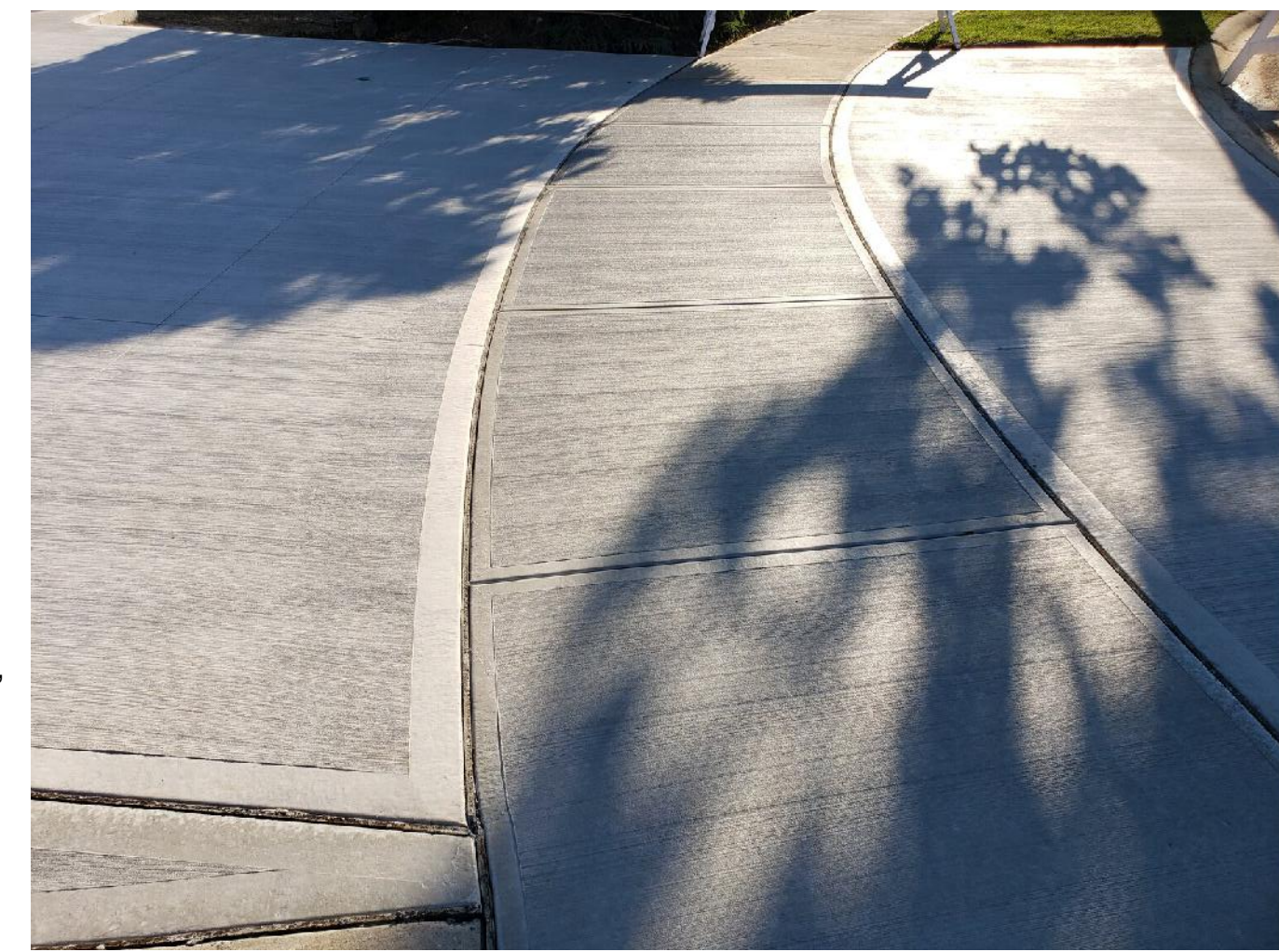
P-101: CONCRETE PAVING CIP CONCRETE | BROOM FINISH | NATURAL GRAY
